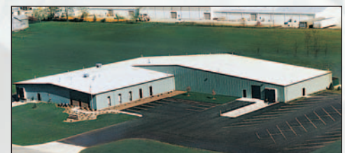
Brookville, Ohio - Manufacturing Plant
