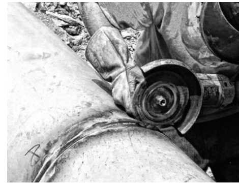
Removing weld slag before the next weld pass.
