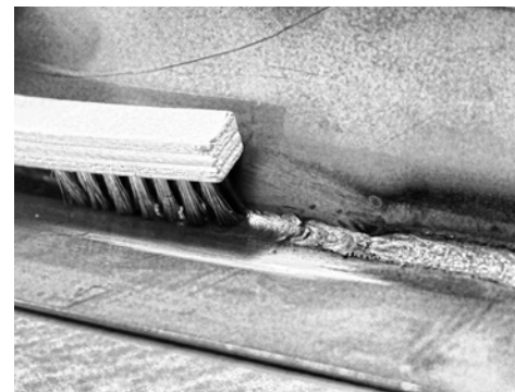
Cleaning a weld with a small scratch brush.
